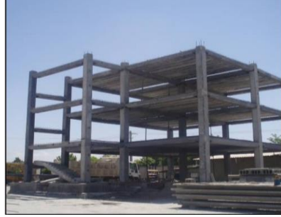
Figure 1, Structural assembling process
